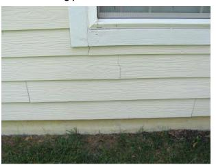
Isolated fiber cement cracks at Unit 500
