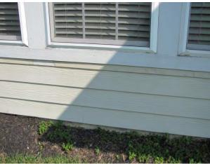
Sealant deterioration and peeling finish at fiber cement, Unit 100
