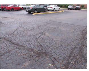
Alligator cracks adjacent to recent patch repair
