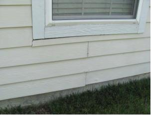
Isolated fiber cement crack at Unit 700
