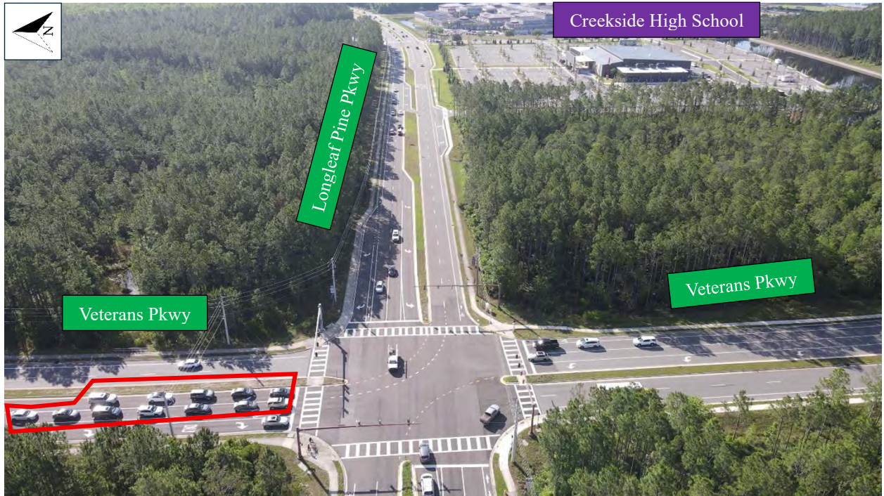
Southbound left-turn queues were observed during AM school peak hour
